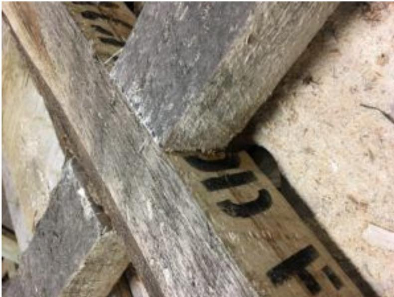
6. Once the joint is secure and not moving, you can then drill a hole large enough for an eye bolt to fit through and secure that with a washer and a bolt.
